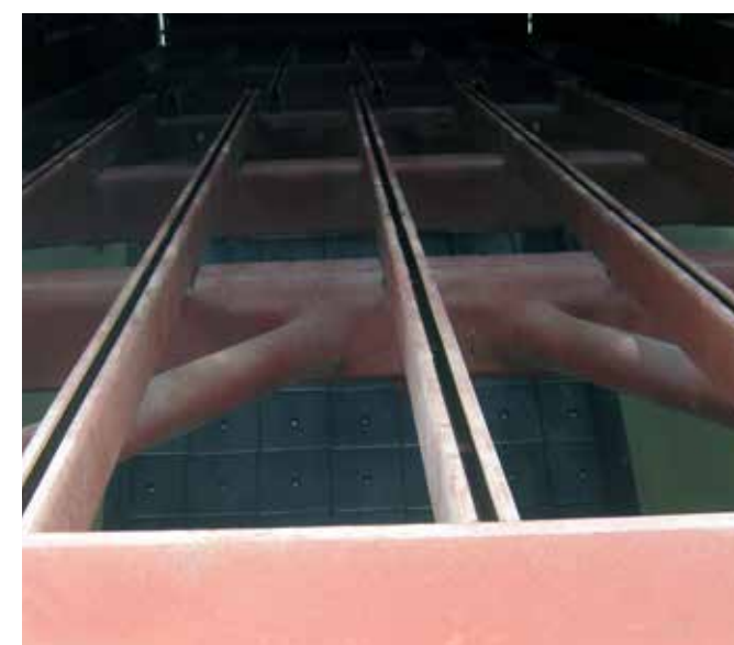
LS-SR rails on construction screen
